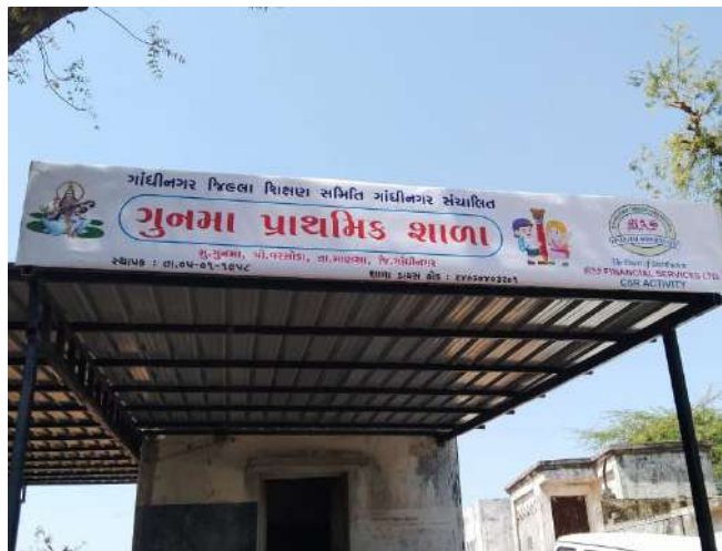
▲ Built School Shed
